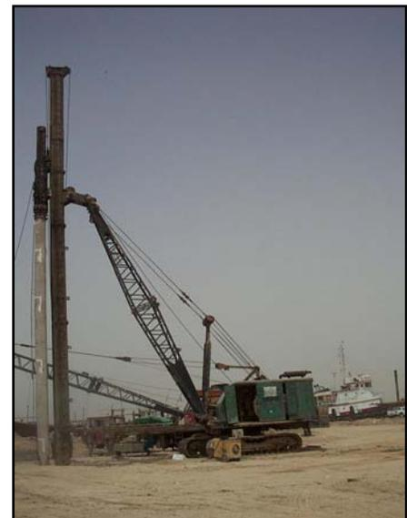
Fig. 3. Pile driving start
