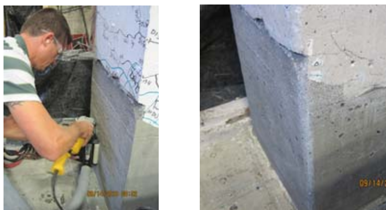
(a) Smoothing Concrete Surface
