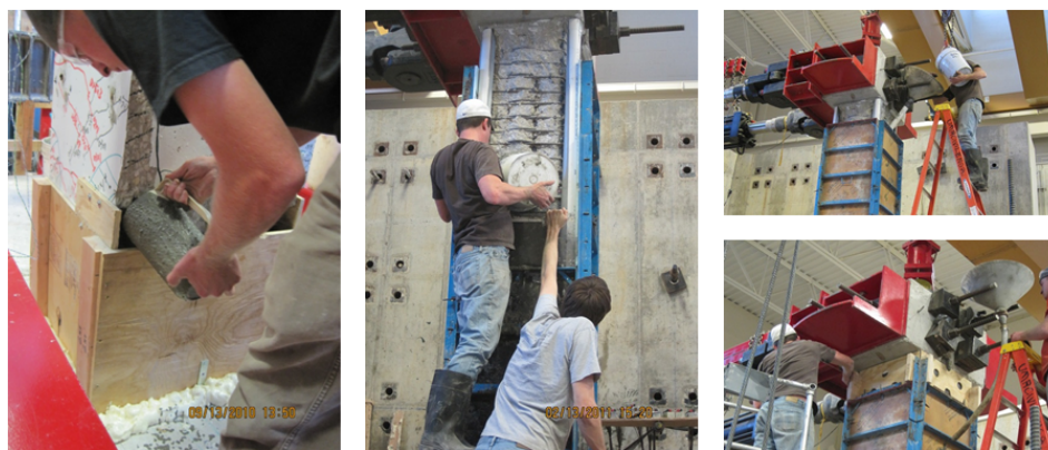
Figure A.4. Placement of Repair Mortar
