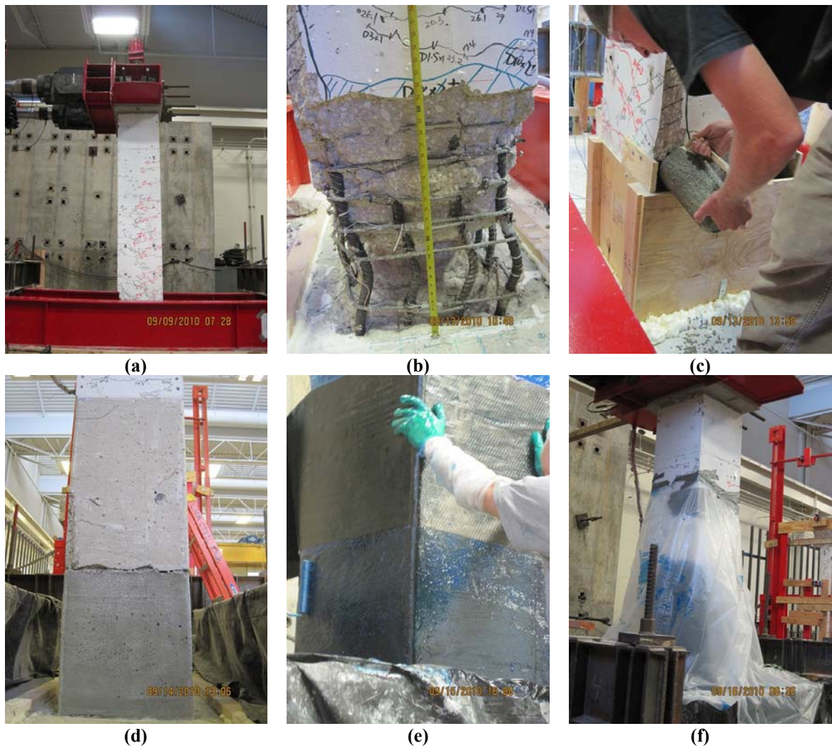
Fig. 11. Repair procedure. (a) Column after straightening, (b) column after loose concrete removal, (c) repair mortar placement, (d) surface preparation, (e) CFRP application, (f) curing process.
