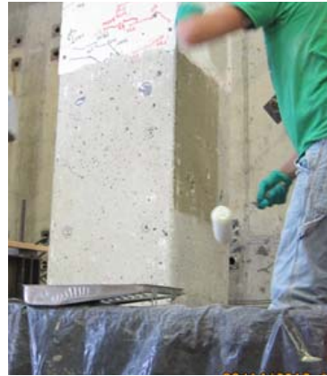
(a) Application of MBrace® Primer
