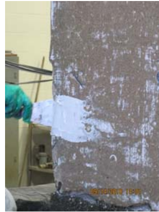
(b) Application of MBrace® Putty
