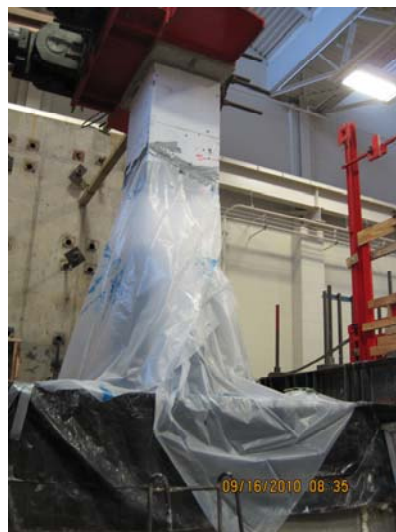
Figure A.8. Curing of the CFRP System
