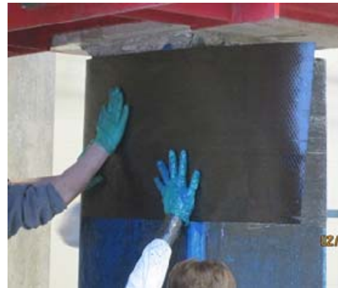
(b) Application of Transverse CFRP
