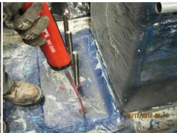
(b) Injecting Epoxy Into Anchor Rod Holes
