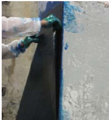
(a) Application of Longitudinal CFRP
