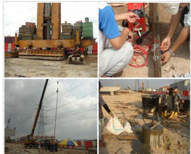
Fig. 3. Typical installation process of spun pile instrumentation in approximate method
