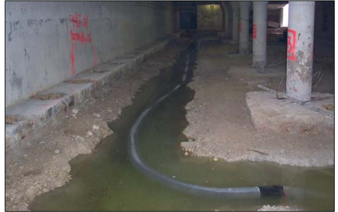
Photograph L – Lateral sock drain installation
