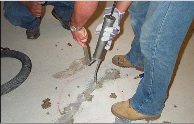
Photograph K – Underslab chemical grouting of joint
