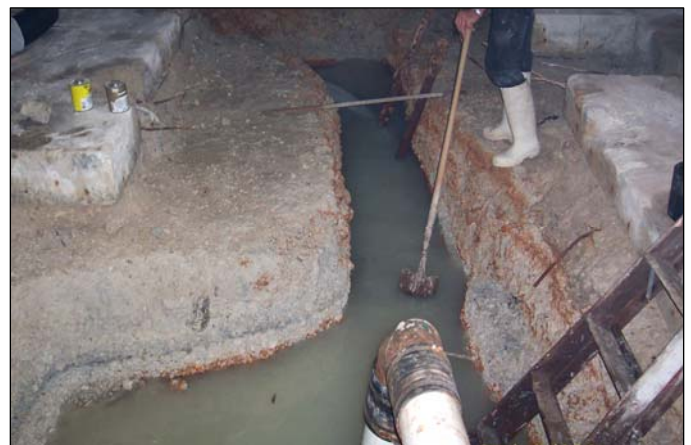
Photograph M – Extraction pit for lateral drain
