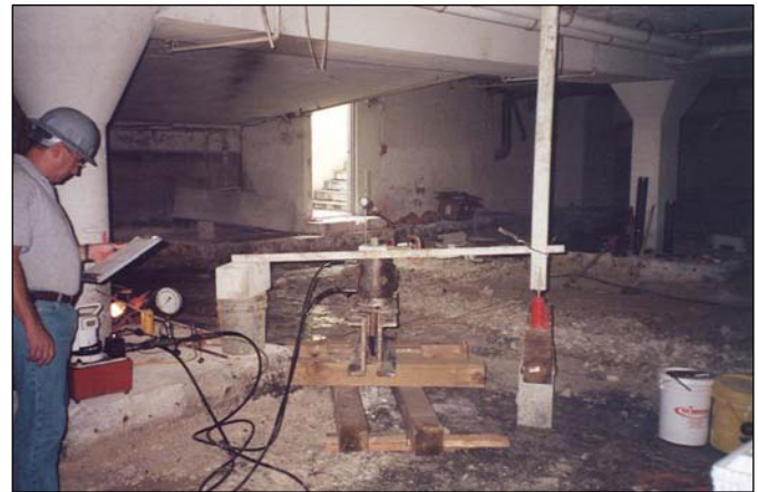
Photograph J – Anchor load test set-up
