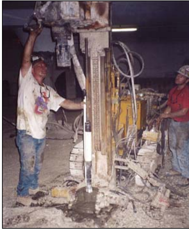
Photograph G – Low headroom anchor rig
