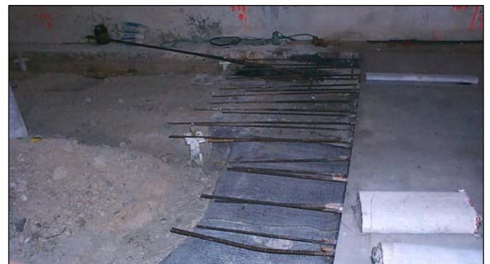
Photograph F – Underslab bentonitic waterproofing
