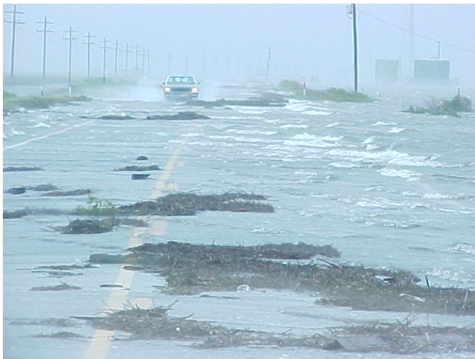
Photograph 1. Condition of the Existing LA-1 during Tropical Storm Bill, 2003)
