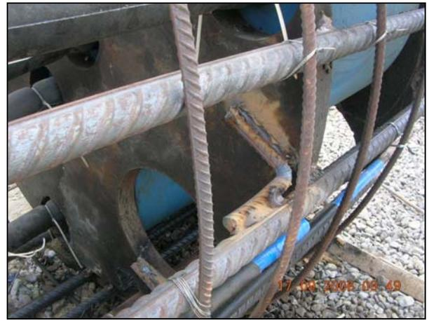
Figure 9: Attaching Steel Plates to the Steel Caging
