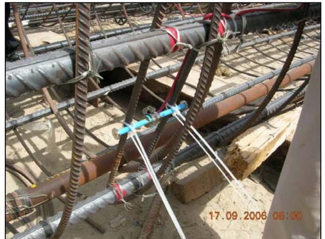
Figure 10: Installation of Vibrating Wire Gauges
