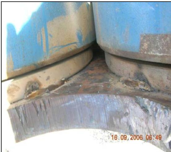
Figure 8: Attaching Steel Plates to the Osterberg Cell
