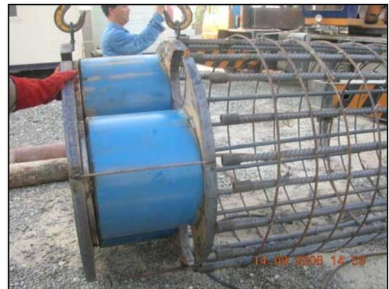
Figure 6: Osterberg Load Cell Installation
