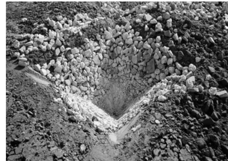
Fig. 7. Typical "Rock Pillar" before up filling
