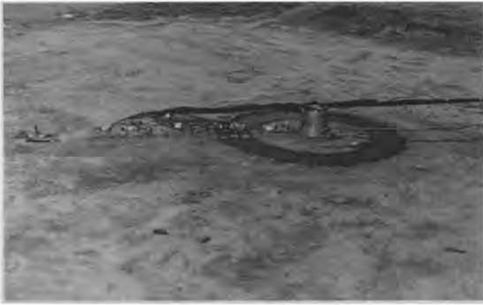
Fig. 8 - Test Setup of Active Isolation by a Soil-Bentonite Trench (Site 1 with barrier)
