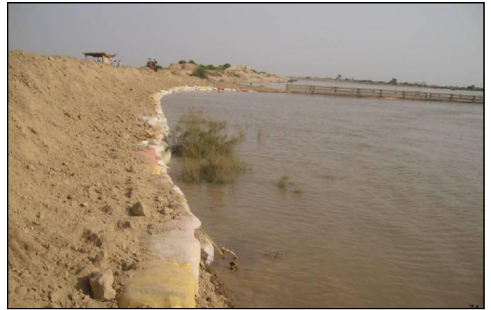
Fig.21 An earthen embankment of RBOD (Amir, 2010)
