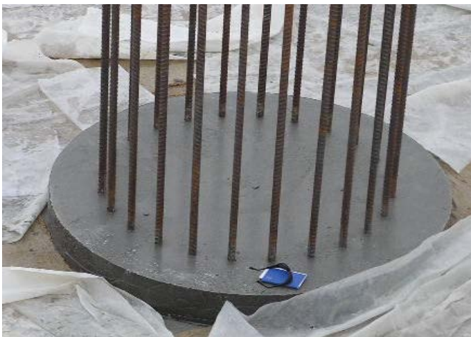
Fig. 7: Pile Head Waterproofing System
