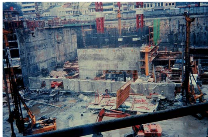
Fig. 18: Plaza Rakyat Office Tower Below-Grade Construction
