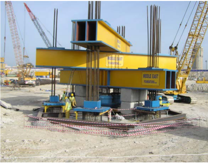
Fig. 6: Pile Load Test
