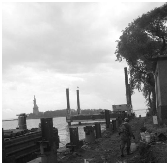
Fig 4. Typical driven piles and seismograph locations with respect to the buildings.
