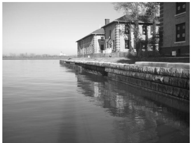
Fig 2. Ellis Island seawalls condition before remedial stabilization.
