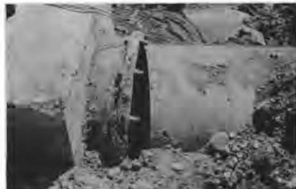
Fig. 5. Damage of Makomanai pipeline.
