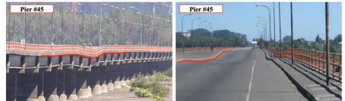
Fig. 8. Liquefaction-induced vertical settlement along the Juan Pablo II Bridge.
