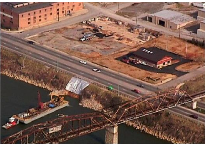
Fig. 4. Air photo taken on 1/22/2003 of tarp covered slide area with orange soil beneath tarp. Note river level on this day varied from Elevation 355.6 to 356.3 ft
