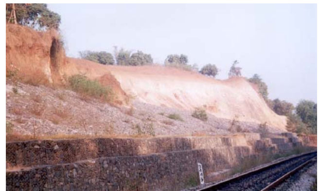
Fig. 2 Construction of Gabion wall along the track
