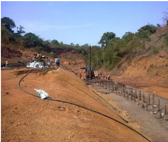
Fig. 3. Construction of Micropiles for the First Bench at RL 25.72.
