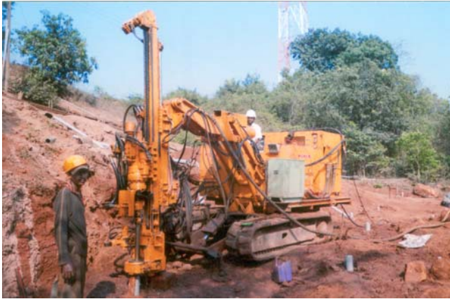
Fig.4. Construction of Micropiles for upper bench and Soil Nails
