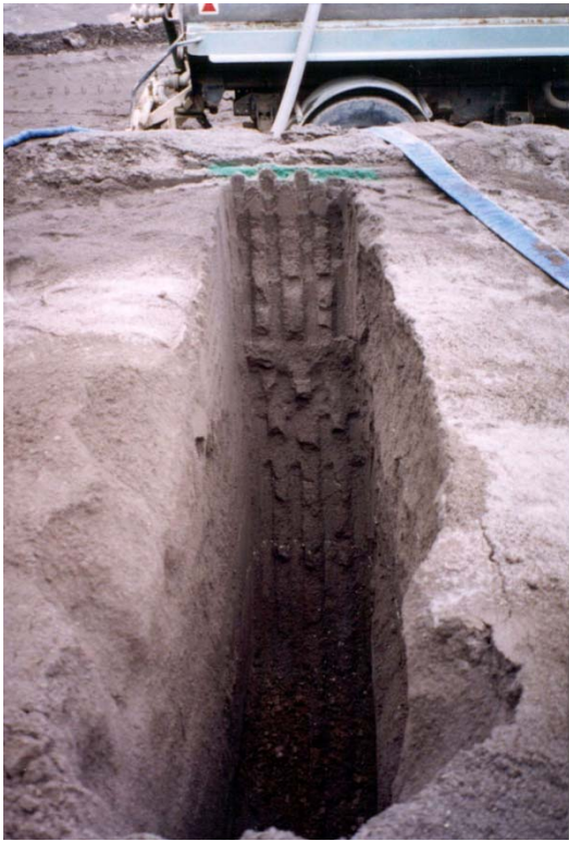
Fig. 6. Trench walls in filter embankment after excavation
