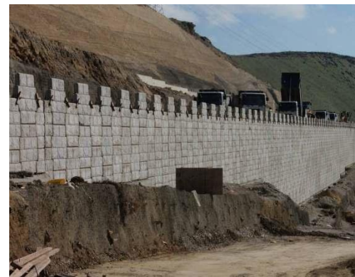
Fig. 10. Construction Phases – Panels and RE Wall
