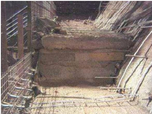
Fig. 5. Friction Connection with Galvanized Steel Ladder Strips
