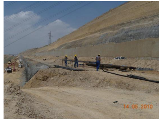
Fig. 6a. Cut Slopes-Drainage and nailing
