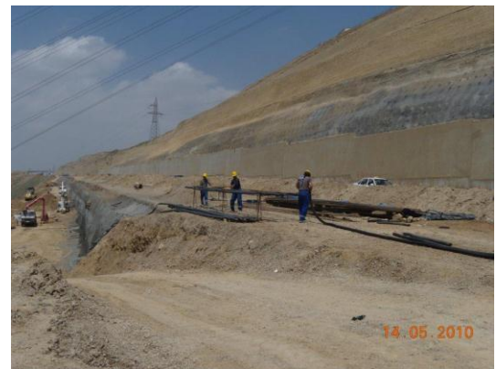
Fig. 6a. Cut Slopes-Drainage and nailing
