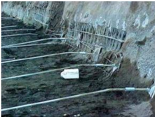
Fig. 4. Direct Connection with Steel Rods
