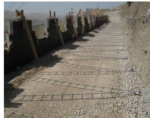
Fig. 9. Construction Phases – Galvanised Steel Ladders
