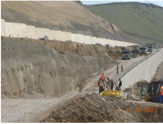
Fig. 7. Linked System Under Construction
