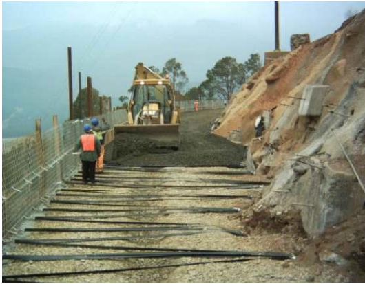
Fig. 3. Direct Connections with Synthetic strips
