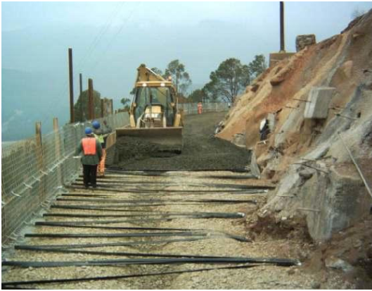
Fig. 3. Direct Connections with Synthetic strips
