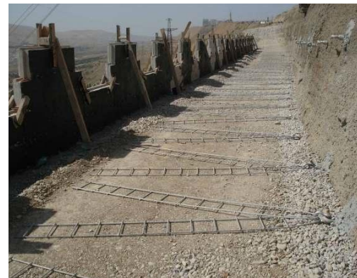
Fig. 9. Construction Phases – Galvanised Steel Ladders
