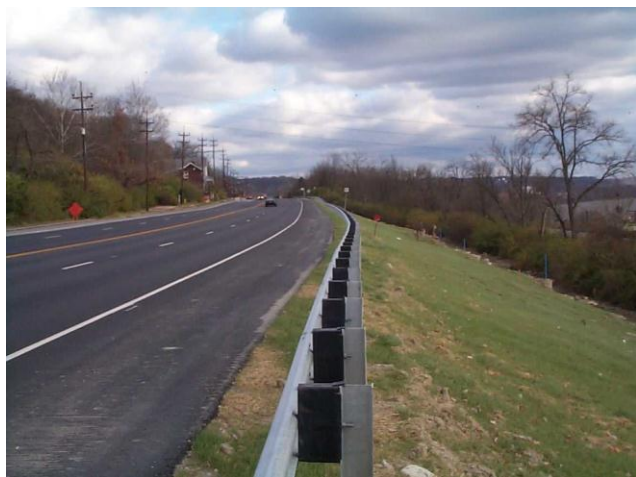
Fig. 17: 2005, after Stub Pier construction.
