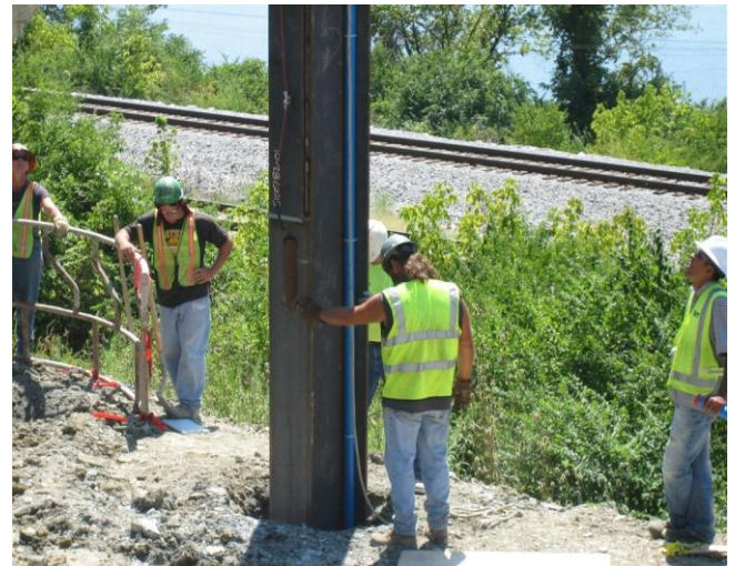
Fig. 10: Setting instrumented steel beam into shaft excavation.
