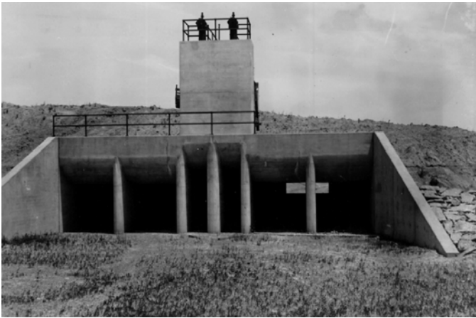
Figure 4 - Conduits Showing Ungated Upstream Inlets Following Original Construction Completion
