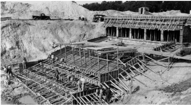
Figure 8 - Outlet Spillway Construction in 1942, Barker Dam
