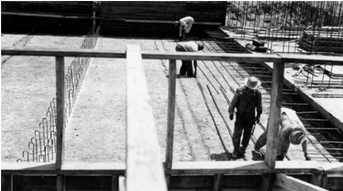
Figure 9 - Outlet Conduit Floor Construction in 1942, Barker Dam
