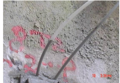
Fig. 15 (c) Exclude air bubbles and bleeding water in process of grouting
