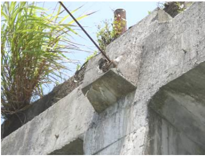
Fig. 9 (a) Tendon fracture and shoot out
