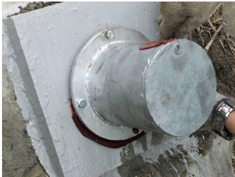
Fig. 16 (d) fixed galvanized cover with bolts Fig. 16 Construction process of corrosion-inhibiting cover
