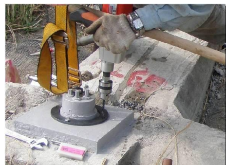
Fig. 16 (a) drilling screw hole on bearing plate
