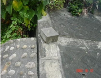
Fig. 9 (b) Depart or rotate of the anchor head
