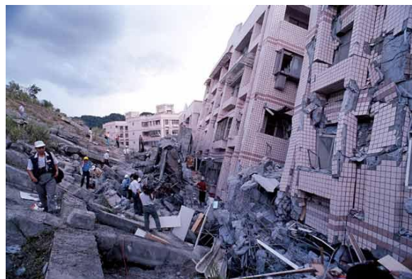
Fig. 8 Landslide of Lincoln Mansion in 1997
