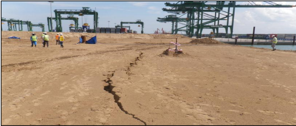
Fig. 1 Downstream view of the first cracks that appeared along the riverbank on April 5, 2010
