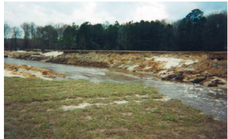
Fig. 5. Photo showing grass surface on spillway.
