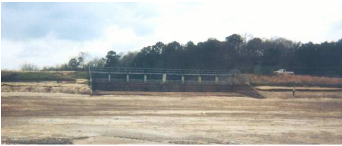
Fig. 6. Photo illustrating principal spillway and typical depth of lake.
