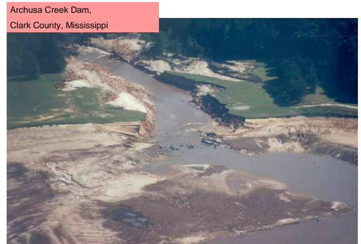
Fig. 4. Close-up view of breach.
