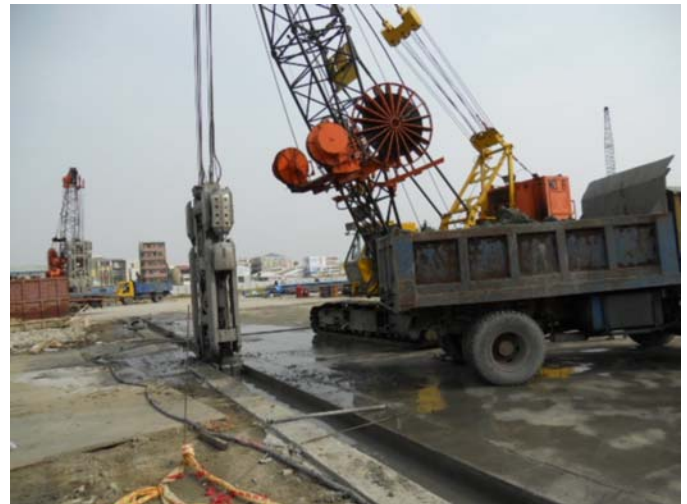
Fig. 15. Installation of Slurry Wall - Tainan
