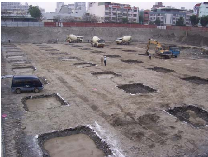
Fig. 8. Footing Excavation – Taichung
