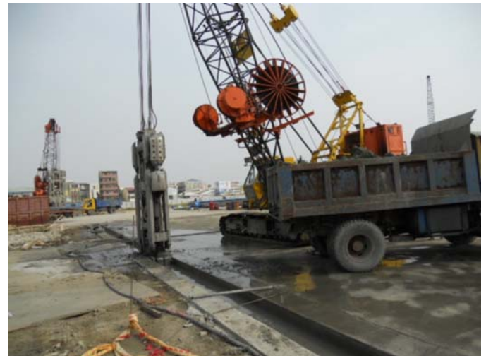
Fig. 15. Installation of Slurry Wall - Tainan
