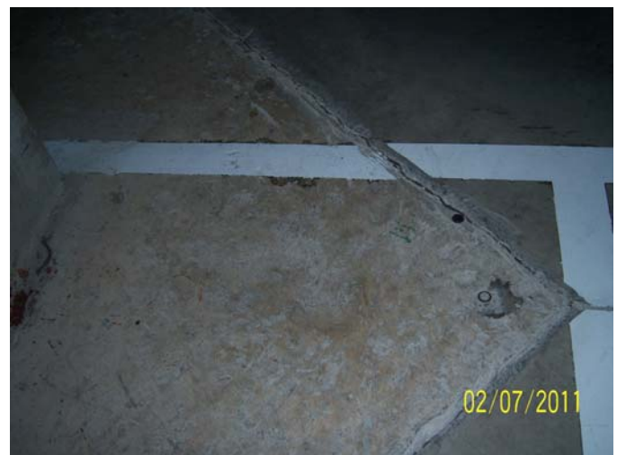
Fig. 9. Repaired Joint - Taichung
