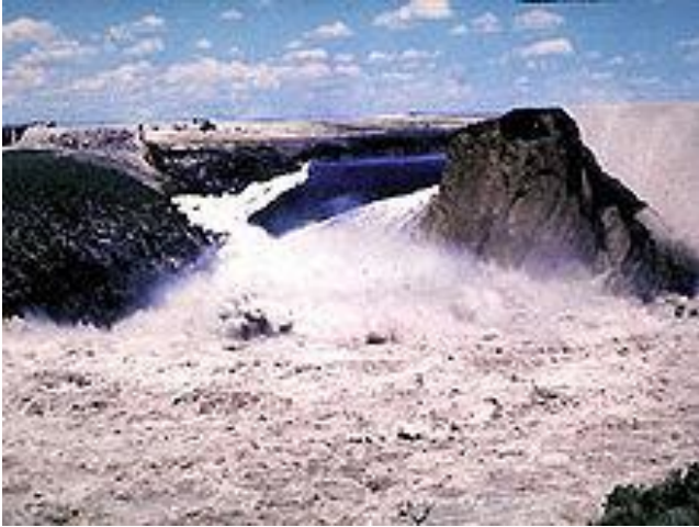
Fig. 4. The Teton dam after failure.
