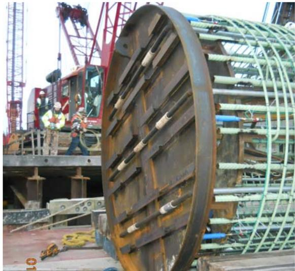
*Fig. 11. Tip grouting apparatus installed at the cage tip.*
