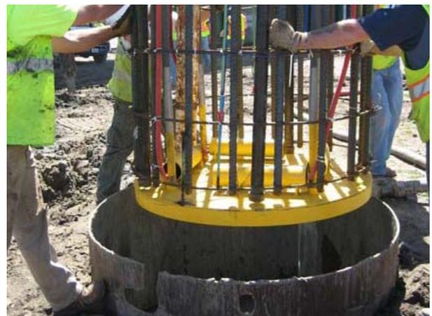
Fig. 5. AFT's tip grouting apparatus being installed in the shaft excavation along with the rebar cage and instrumentation
