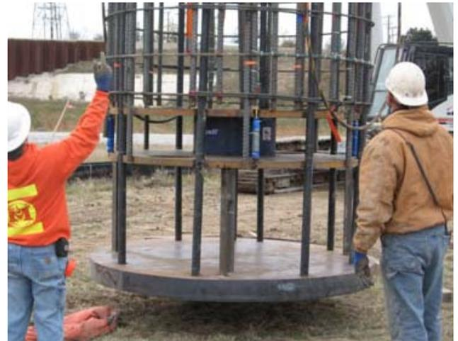
Fig. 7. O-cell and tube-a-manchette system in rebar cage
