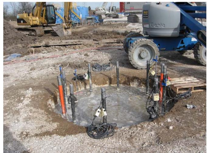
Fig. 8. Installed Test Shaft CTS-1
