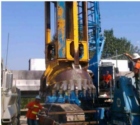
Fig. 3. Malcolm Drilling's clam shell grab
