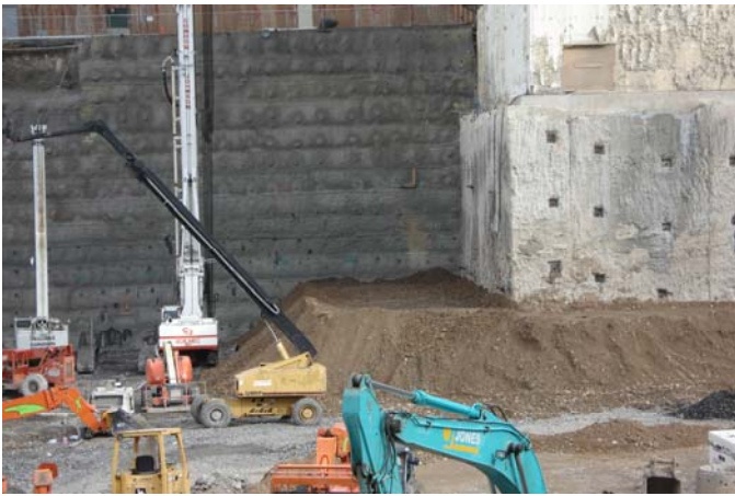
Fig. 5. Stabilizing Berm
