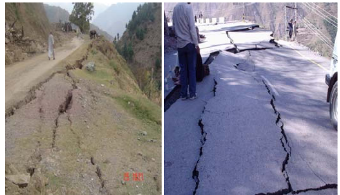
Figure 15. Longitudinal cracks on roads aligned parallel to slopes.
