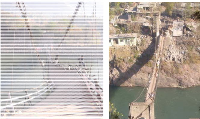
Figure 19. Damage to suspension bridges.
