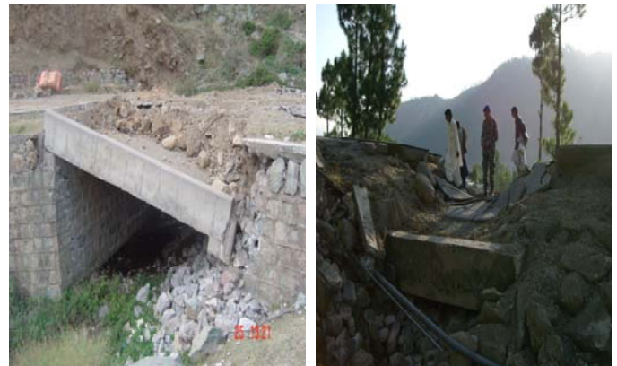
Figure 16. Most of the culverts in most affected area were damaged.
