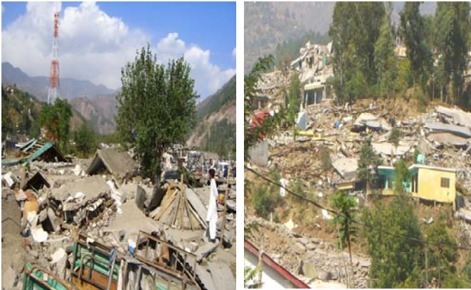
Figure 7. Masonry buildings on slopes were razed to ground in Balakot area.
