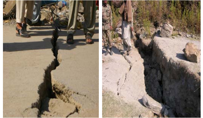
Figure 14. Transverse cracks on roads showing tension cracks.
