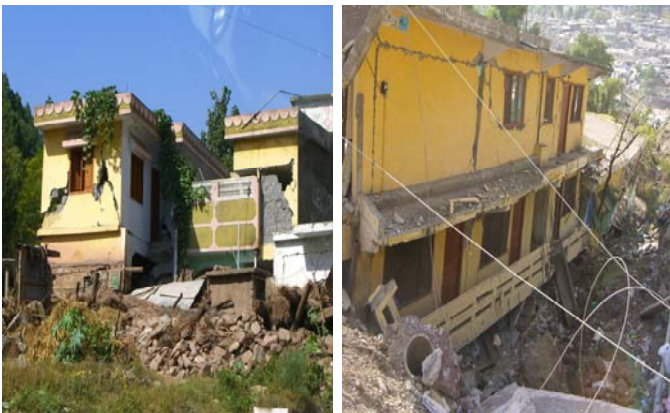
Figure 9. Some buildings with relatively better construction though damaged but withstood the earthquake shaking.
