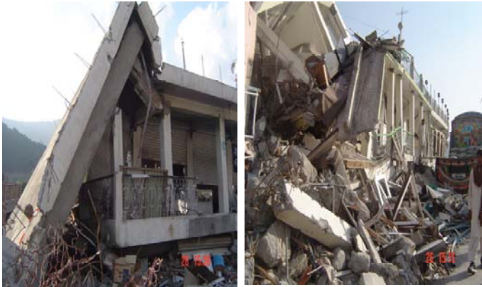
Figure 10. Visible reinforcement; an indication of very poor construction practices.
