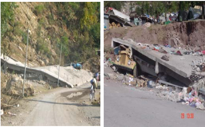
Figure 8. Concrete buildings with poor foundation and construction were collapsed in Balakot area.
