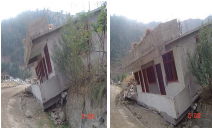
Figure 11. A building displaced laterally but stayed intact; an evidence of good construction.
