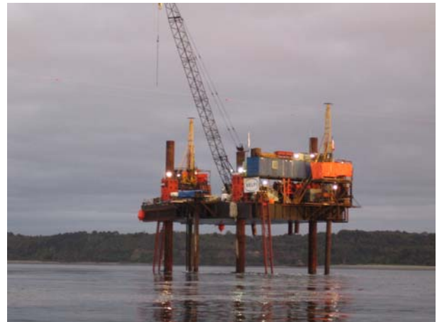
Fig. 7. Jack-up Platform on top of Roca Remolinos
