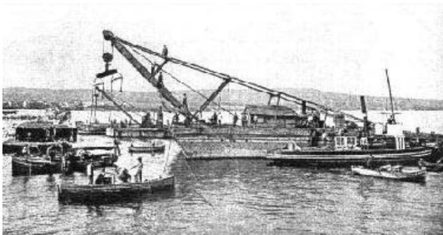
Fig8. Floating crane for the stone blocs (1896-1903)
