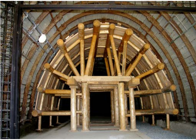
Fig.5. Replica of wooden support system
