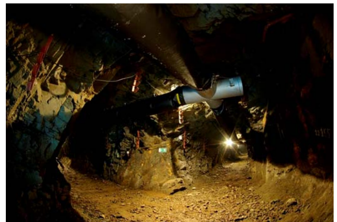
Fig.4. View of a gallery intersection during reconstruction
