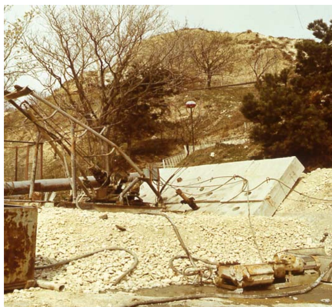
Fig.5. Construction of pre-strained anchors in Balchik (1988)
