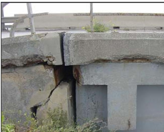
*Photo 3. Rotation of approach slabs followed by structure damages.*
