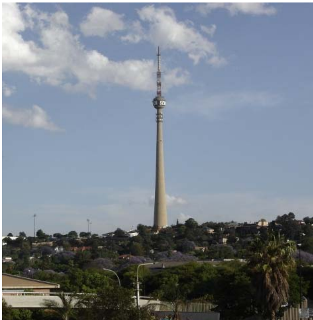
Fig. 2. The Sentech Tower (2007), completed in 1961, formerly known as the Albert Hertzog Tower and Brixton Tower consecutively (photograph Lizè Groenewald).
