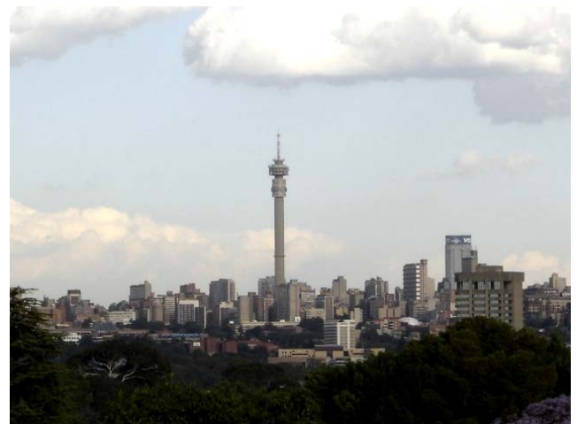
Fig.3. The Telkom Joburg Tower (2007), completed in 1971 and formerly known as the JG Strijdom Tower but informally called the ‘Hillbrow’ tower until 2005 (photograph Lizè Groenewald).
