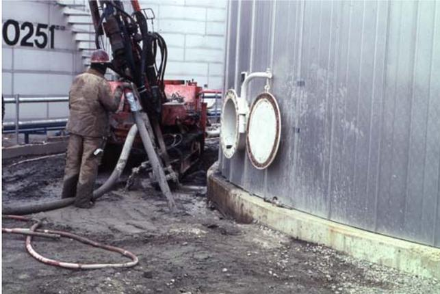
Fig. 11. Remedial grouting programme in progress
