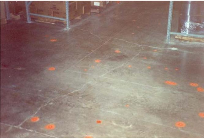
Fig. 4. Warehouse slab exhibiting transverse cracking and popouts (painted orange for identification purposes).
