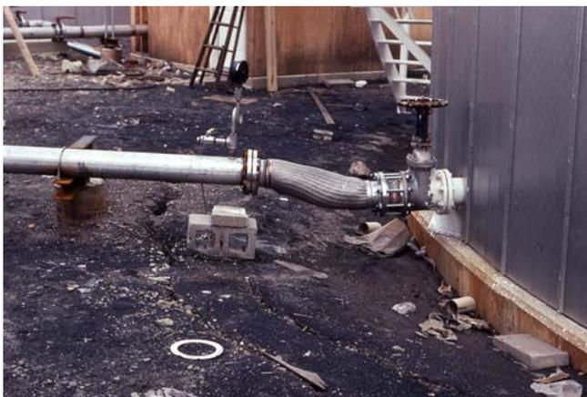
*Fig. 8. Flexible connection indicates movement and ground failure*
