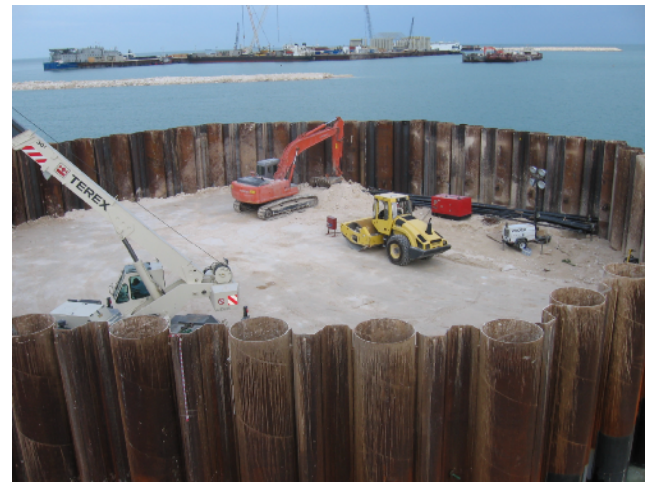
Fig.16. Steel pipe pile driving works at Barrier Head
