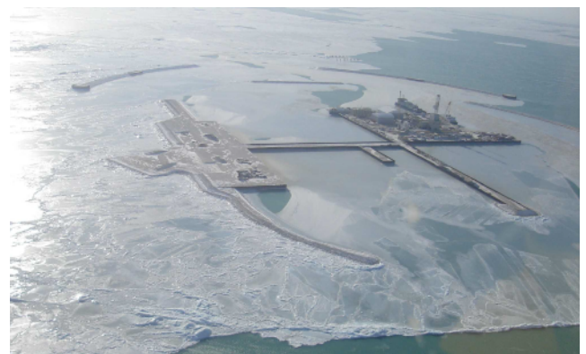
Fig.8. Ice ridge around the trial cofferdams at D-Island Complex
