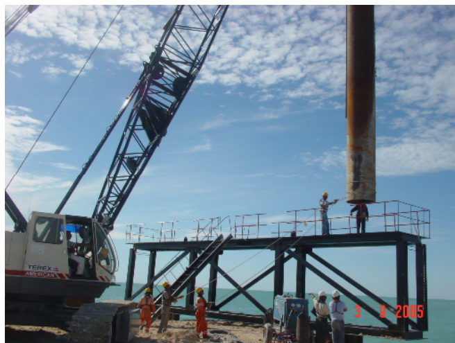
Fig.12. Specially manufactured steel guide frame
