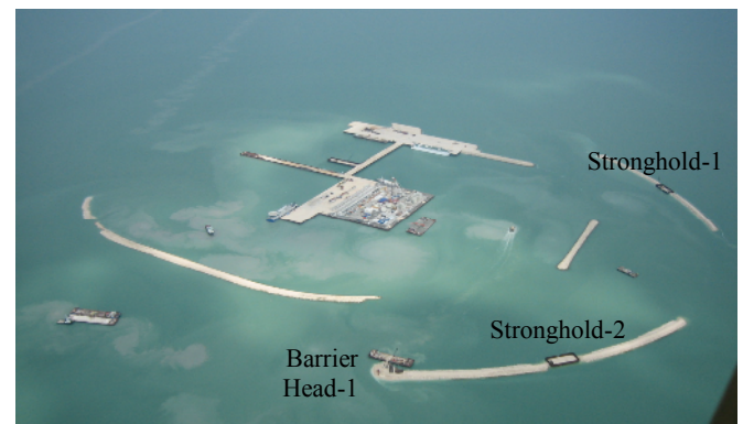
Fig.7. Trial cofferdams at the D-Island Complex
