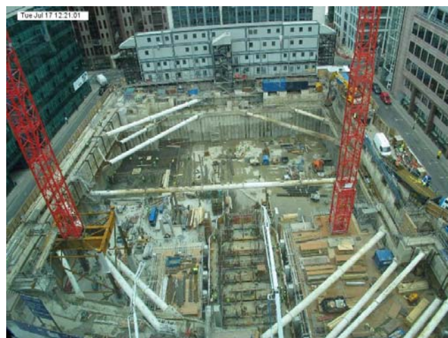
Fig. 25. Excavation at formation level of the basement of the Ropemaker Project
