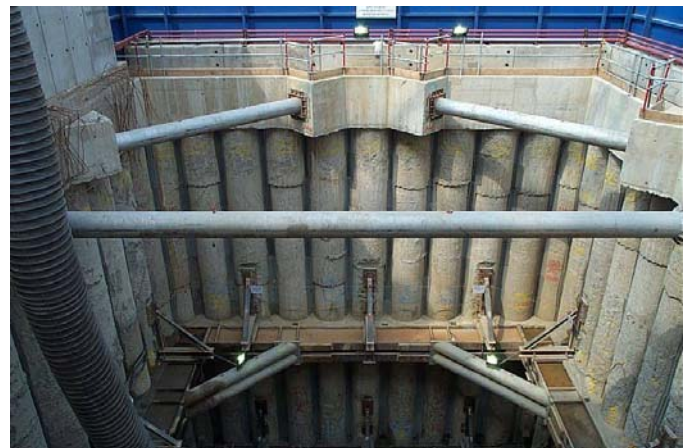
Fig. 16. Image of the excavation at Kings Cross Hub Shaft
