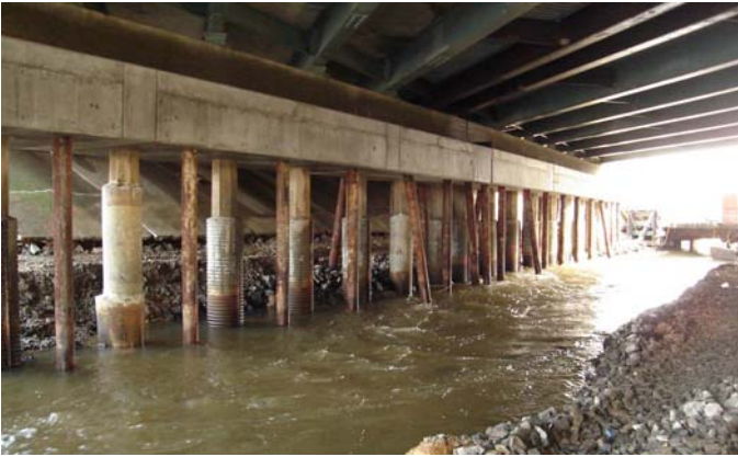
Fig9. View of micropiles and completed cap beam.
