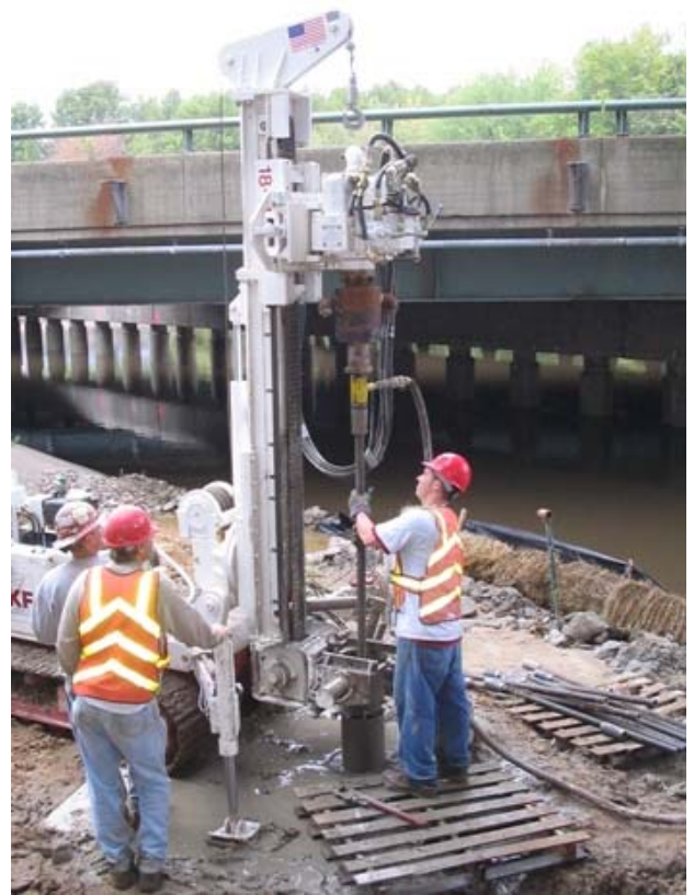
Fig. 4. Drilling of test hollow core bar micropile through casing.
