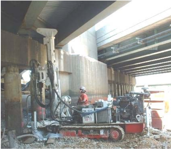
Fig. 3. Installation of production micropiles with limited headroom.
