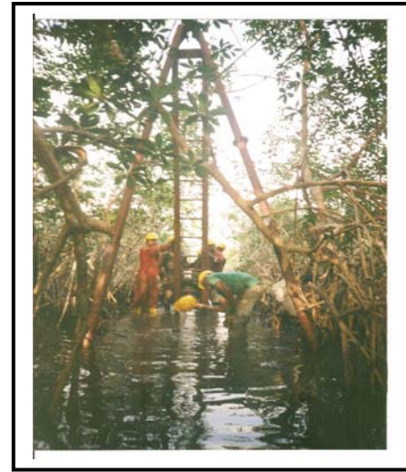
Fig. 3. Percussion Rig used at the Bridge Abutment Sites.
