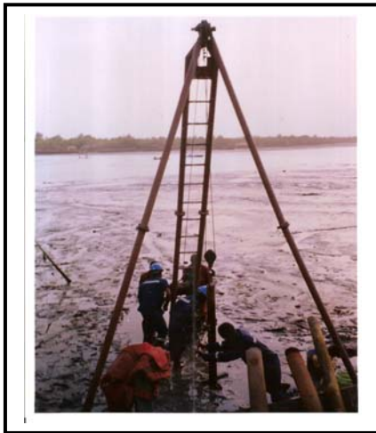
Fig. 3. Percussion Rig used adjacent to the Building Sites.
