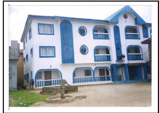
Fig. 7a. Frontal view of the two-storey building leaning backwards.
