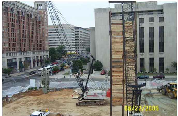
Fig. 6. Setting of Prefabricated Panel.
