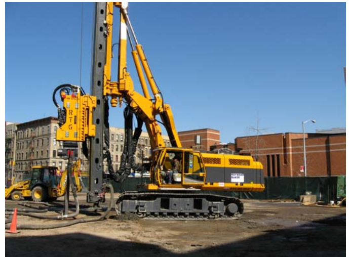
Fig. 5. Photograph of Grout Casing Installed to Approximately 45 ft depth.
