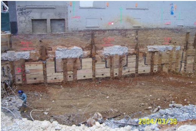
Figure 6: Existing Bracket Piles Supporting 1899
