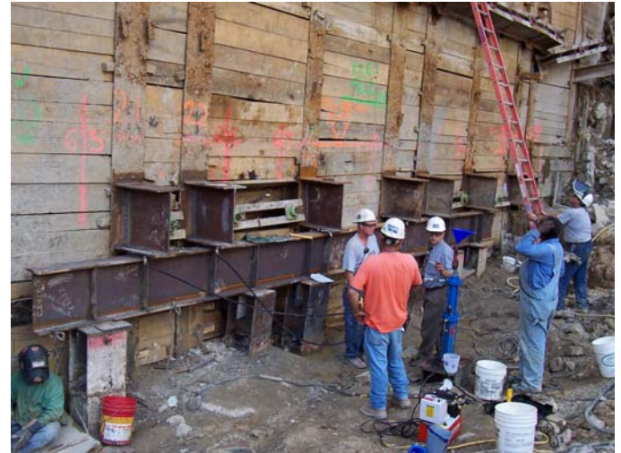
Figure 12: Three Brackets Pre-stressed Simultaneously
