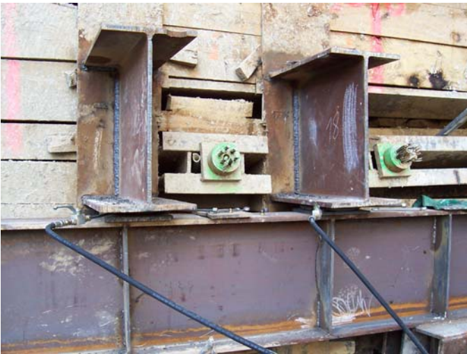
Figure 11: Completed Lower Jacking System
