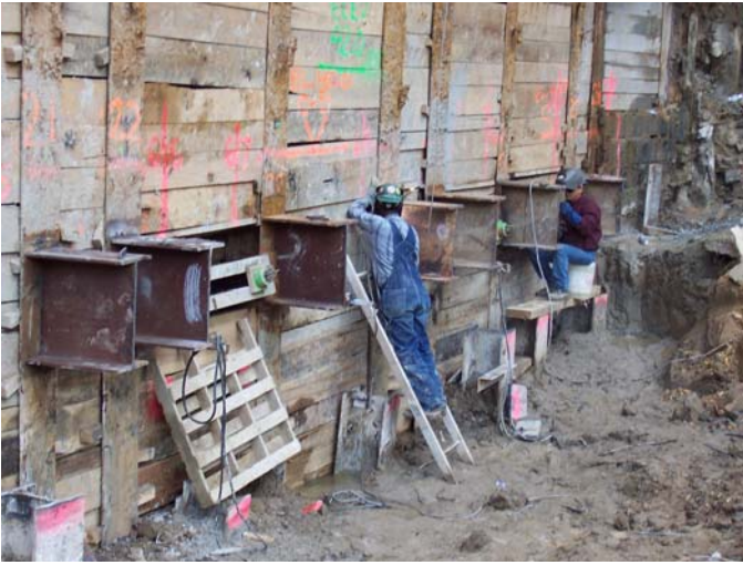
Figure 10: Installing lower brackets
