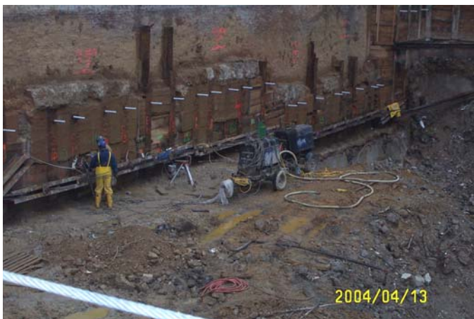
Figure 8: Testing Top Tier Tiebacks & Old Foundation Wall (to be removed)
