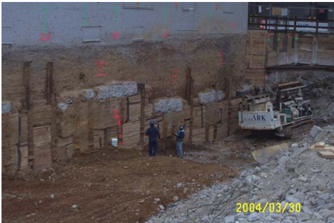
Figure 7: FBE-2T Drilling Top Tier Tiebacks
