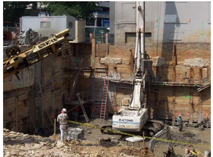
Figure 9: SoilMec Installing New Bracket Piles
