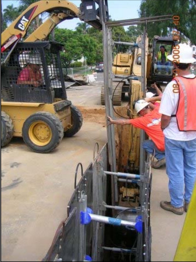
Fig. 6. Sequential shoring operations in fast-raveling sands.
