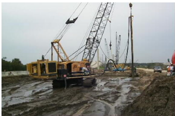
Plate-3: Stone Column by Vibro-replacement Method
