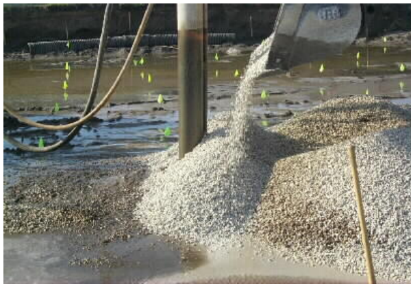
Plate-4: Stones being poured into the Drilled Shaft
