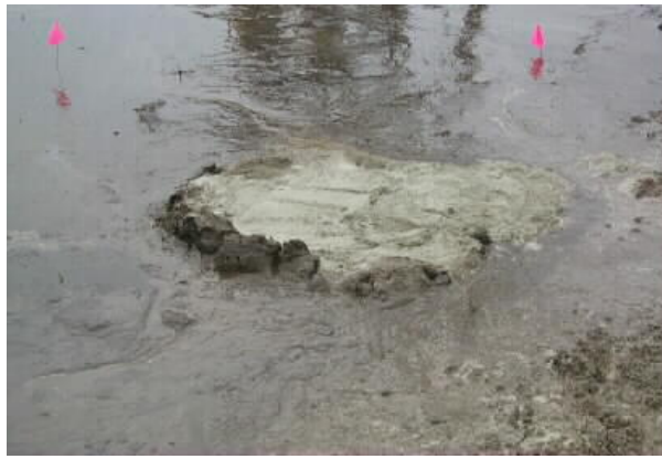
Plate-5: Finished Stone Column
