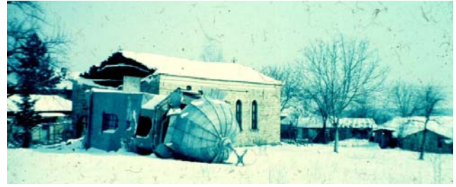
Fig. 4. Destroyed church tower in Mirovo village (Gorna Oryahovitza's zone) during the earthquake with magnitude M=5.1 (February 1986) [Shanov S., 2006]
