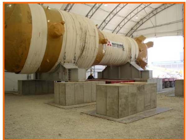
Fig 2. Storage facility with one steam generator in place
