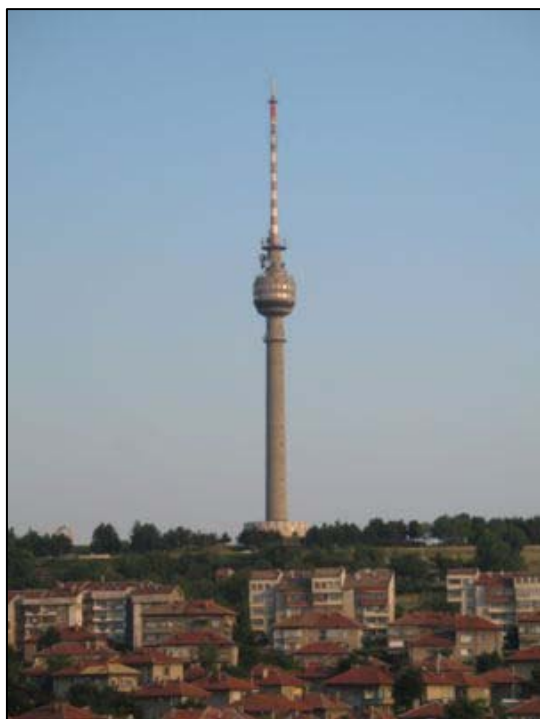
Fig. 1. General view of the TV tower in Rouse city
