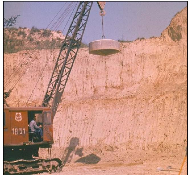
Photo 1. Heavy tamping of the excavation bottom - L<sub>1</sub>, FS<sub>1</sub>, L<sub>2</sub> and FS<sub>2</sub> can be distinguished on the vertical slope
