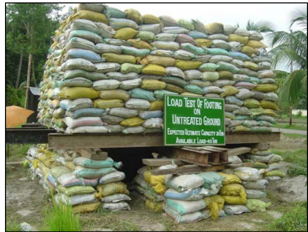
Fig. 5. Set up of load arrangement for footing load test.
