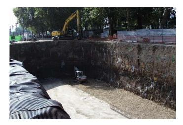
Before the recommendation of a superficial protection of the court before the atmospherically agents, is adopted the placement of a drainage plate, of whose placement is deduced its void functionality as waterproof you, to indicate that was not put any perimeter drainage of the joint.
