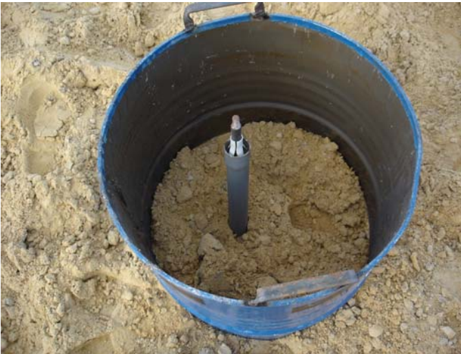
Fig. 15. Installed settlement plate.
