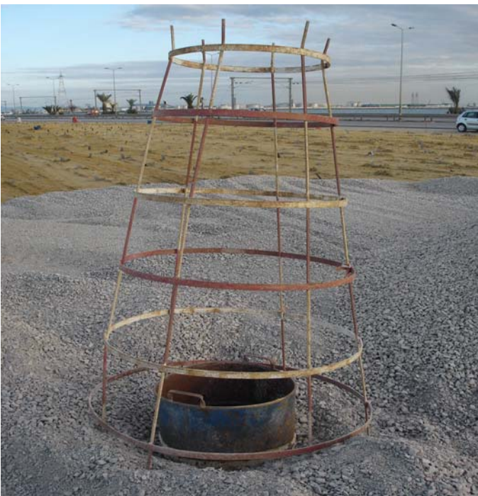
Fig. 16. Protected settlement recorder.
