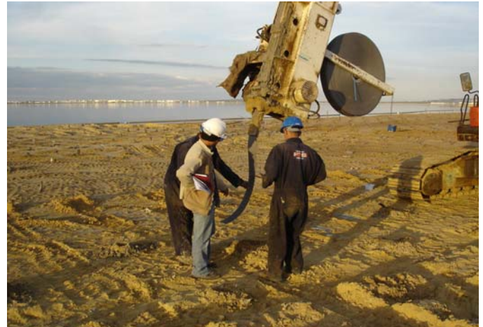
Fig. 13. Starting PVD installation.
